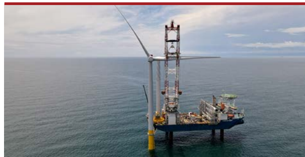
ONE UP: Jan De Nul jack-up Vole au Vent installed the first Siemens Gamesa 6MW turbine at Coastal Virginia last week. First power is expected late summer or early fall.
