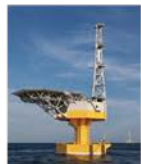
"Fukushima Kizuna" The World's first floating substation
