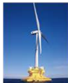
"Fukushima Hamakaze" 5MW Floating wind turbine
