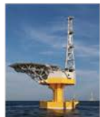
"Fukushima Kizuna" The World's first floating substation
