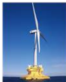
"Fukushima Hamakaze" 5MW Floating wind turbine
